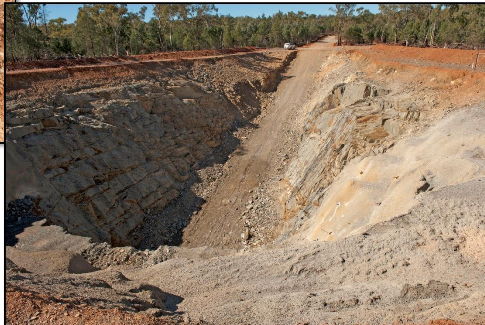
Hera Boxcut Complete
