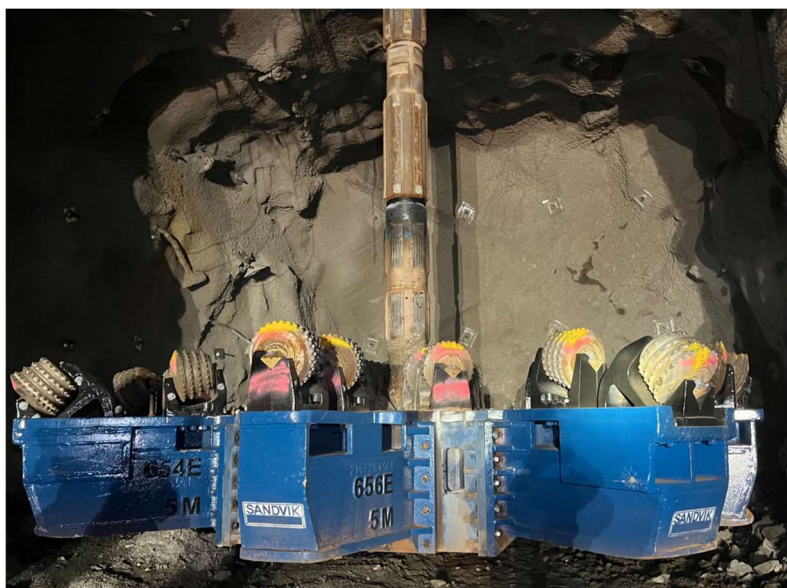
Image 2: Reamer head ready to commence reaming the return air raise (RAR).
