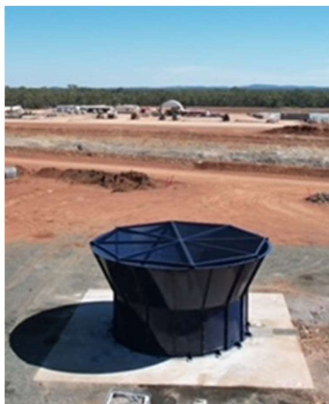
Image 3: Fresh air raise (FAR) evase in place.
