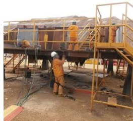
On-site maintenance and shutdown services (Pilbara Hire)
