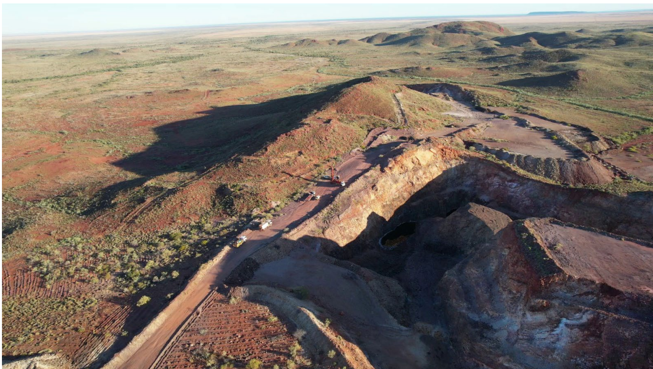
Figure 2: TopDrill Mobilisation to Whim Creek Copper Project
