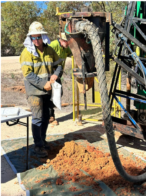
Figure 3: Parrakie aircore drilling Loxton/Parilla Sands (left) and clay/clayey sands intersected in the drilling
