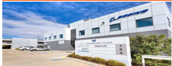
1 and 2 Technology Place Williamtown, NSW
