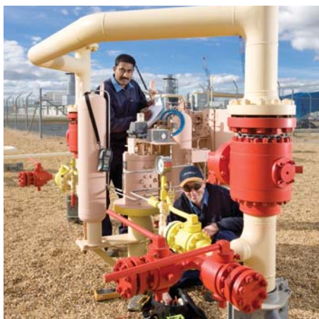
Satya Nand and Mick Mara servicing the mainline valve which feeds gas into Origin Energy's power station, Uranquinty, New South Wales
