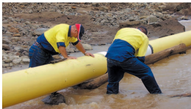
The exposed Rocky Creek RBP 16" transmission line at the base of the Toowoomba Range is normally buried more than under 1.2 metres underground.
