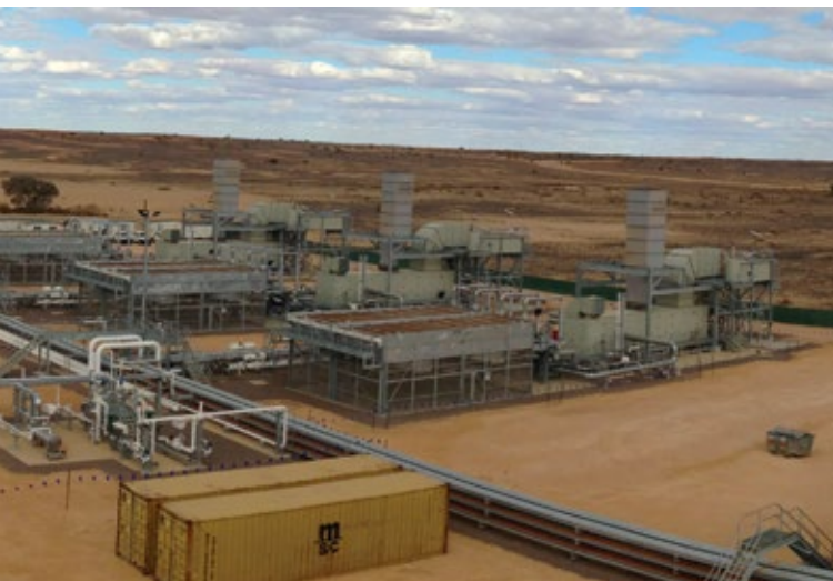
Expanded compression capacity at Moomba with the installation of 3 new Solar Mars 90 compressors.
