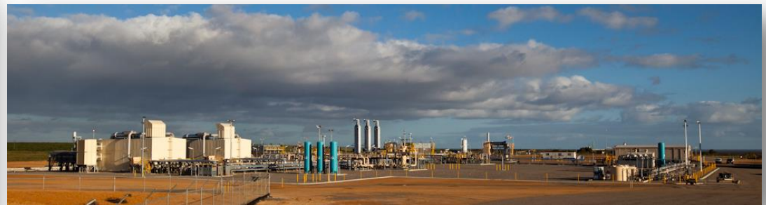
Mondarra Gas Storage Facility
