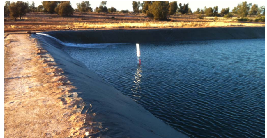
Pilot evaporation ponds prior to final commissioning
