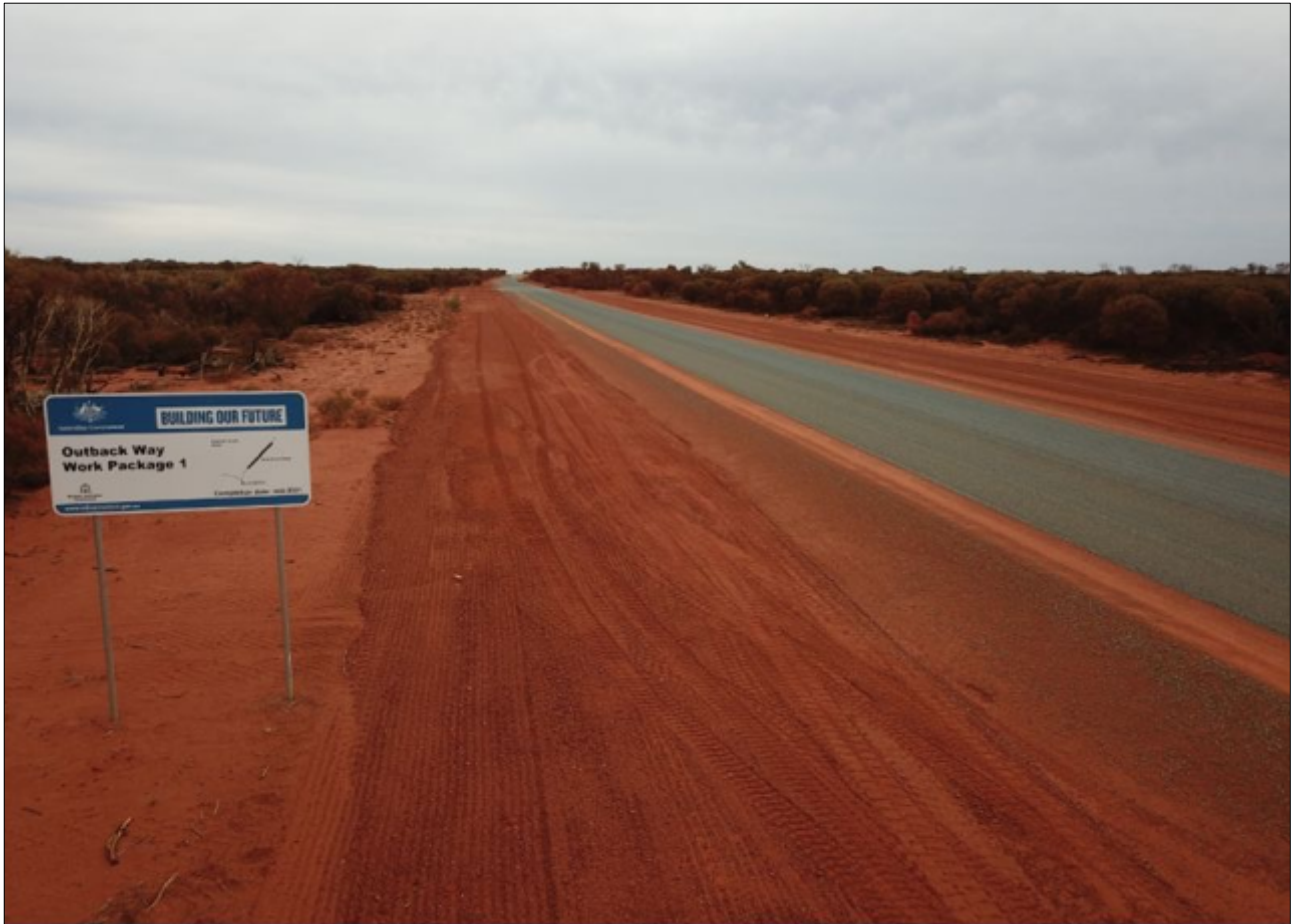
Figure 12 Great Central Road Surface Sealing Program
