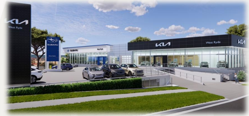
Ryde Kia & Ryde Subaru, Sydney – Under Construction
