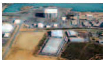
Trailcraft Industrial Complex 99 Quill Way, Henderson, Western Australia
