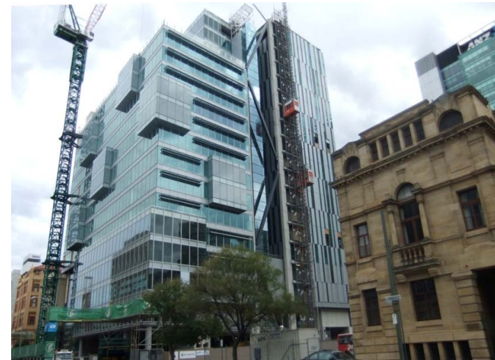
ATO Building under construction, Adelaide
