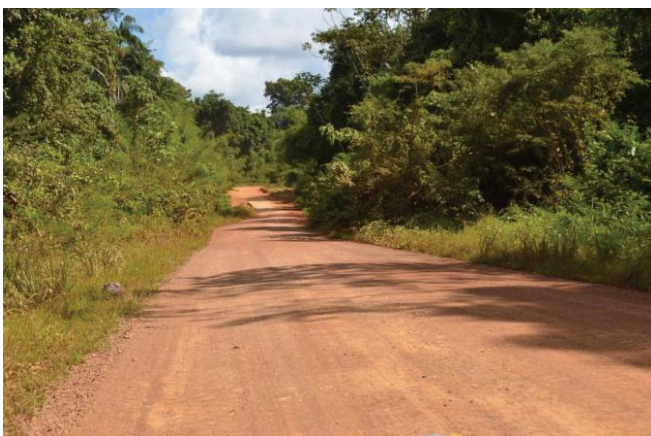
Figure 4: Access road at Arakaka
