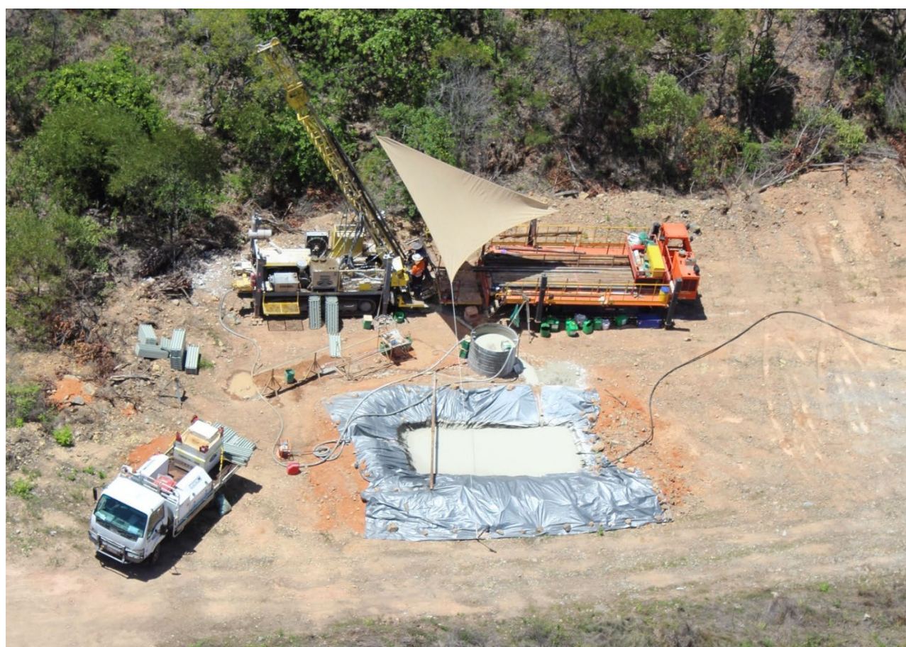
Figure 1. Previous diamond core drilling at Horn Island
