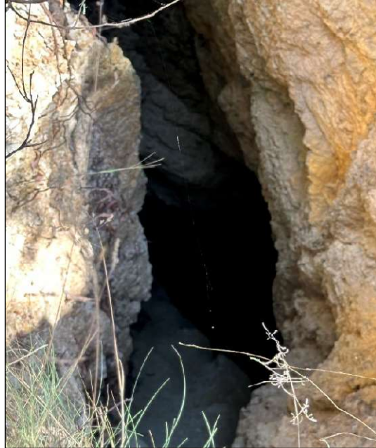
Figure 2 – Vertical shaft/stopes. Located at 711647E, 6258732N.
