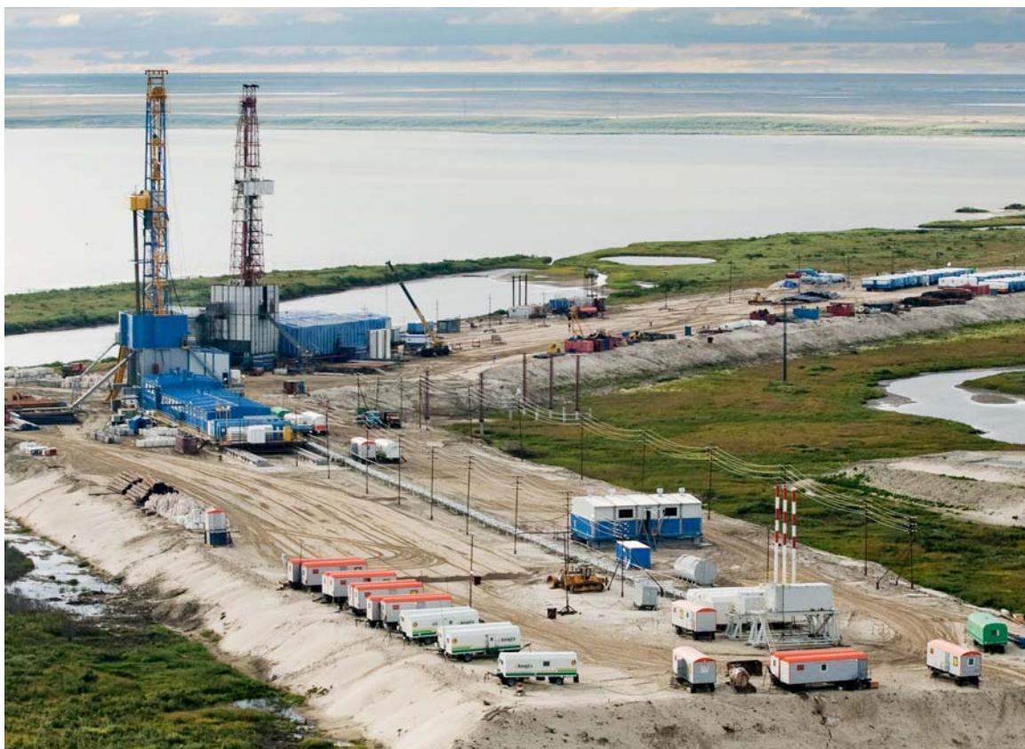
PRODUCTION DRILLING AT THE YURKHAROVSKOYE FIELD
