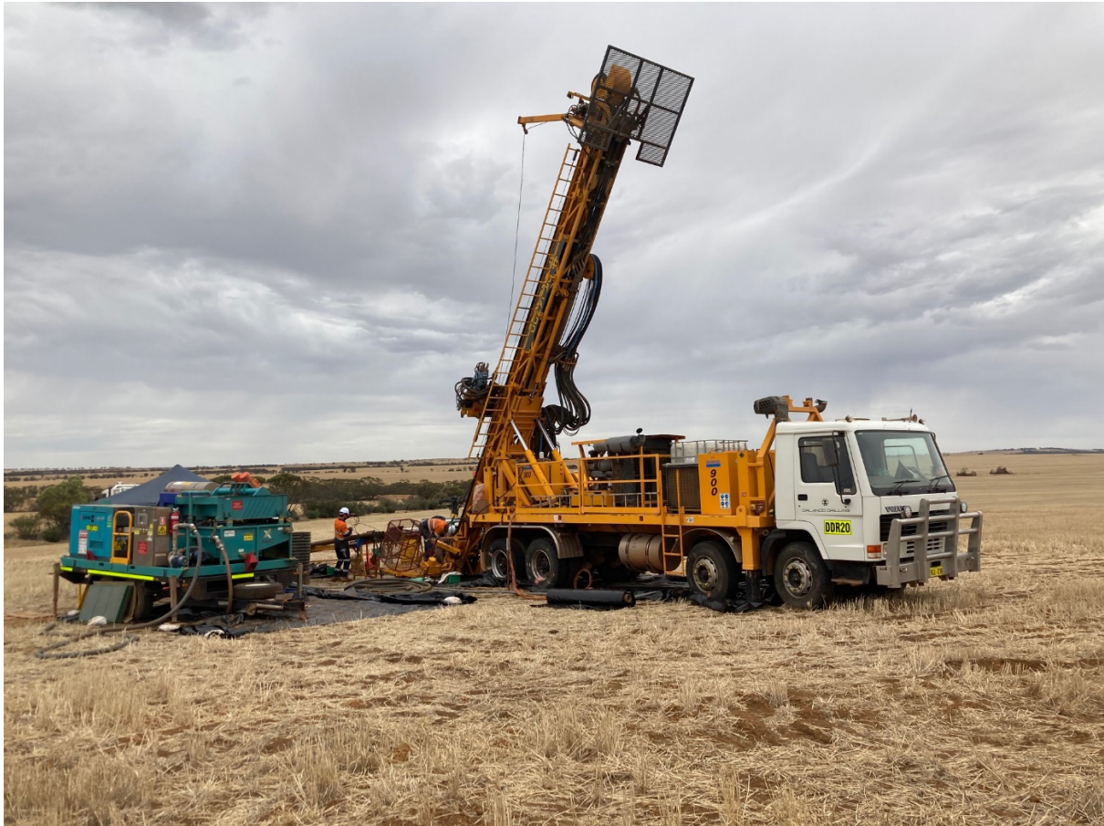
Figure 1. Orlando Rig DDR20 at work.
