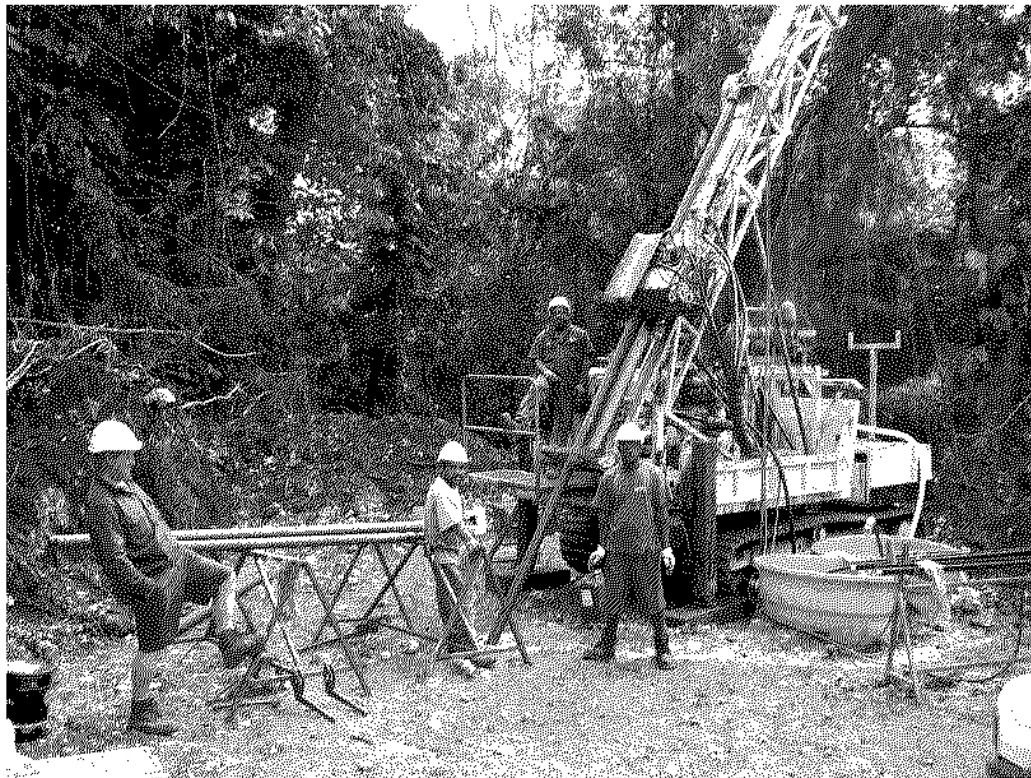
Alcaston drilling at Webe Creek in Vanuatu
