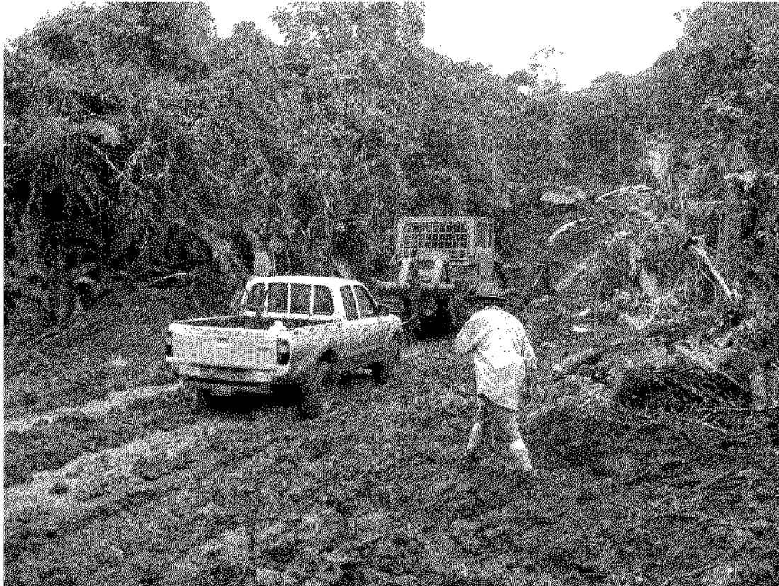
Newly constructed access road at Webe Creek in Vanuatu. Unseasonal rain has hampered the drilling program.
