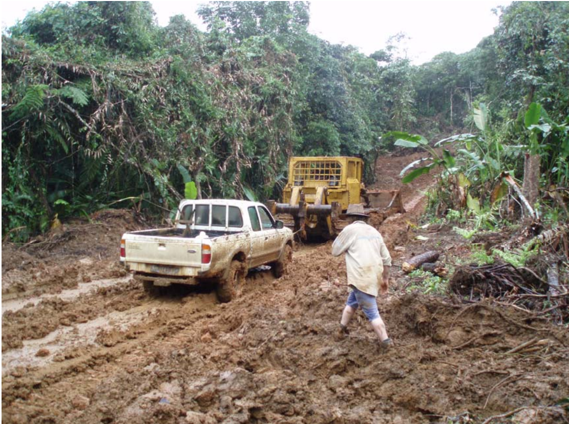
Newly constructed access road at Webe Creek in Vanuatu. Unseasonal rain severely hampered the drilling program.
