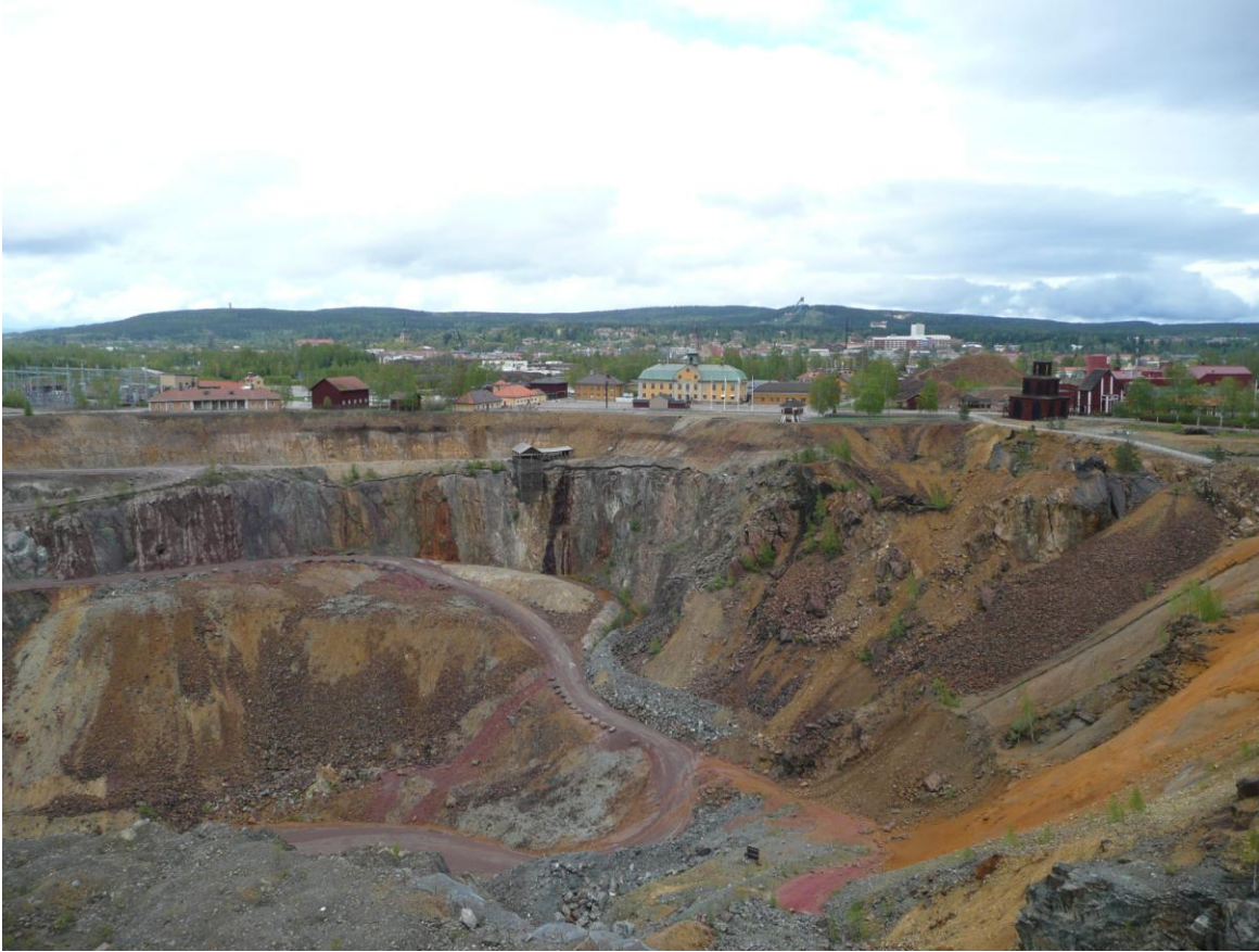
Photograph 3. The Falun open pit in central Sweden. A major underground mine extends beneath this pit to a depth of around 500 metres.
