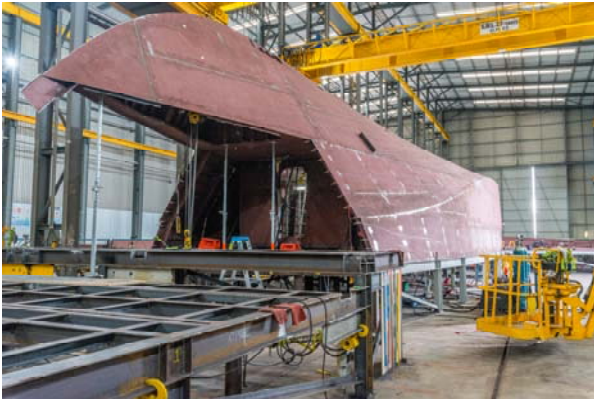
Pacific Patrol Boat Replacement (PPB-R) under construction at Austal Australia
