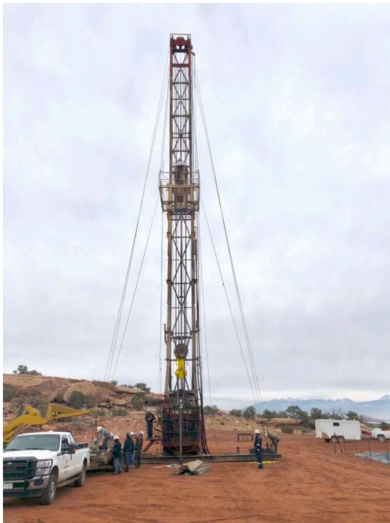
Figure 1: Drill rig set up on site.
