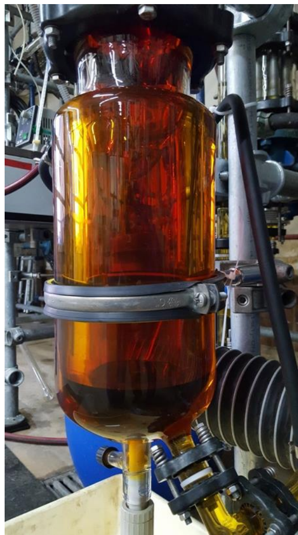
Figure 3: Reboiler with Bromine
