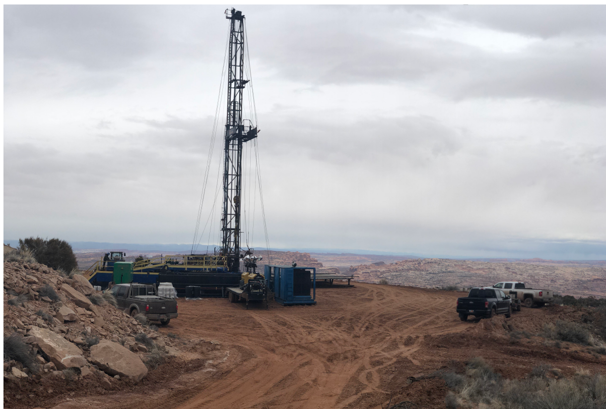
Figure 1: Drill Rig at the Long Canyon No.2 Well
