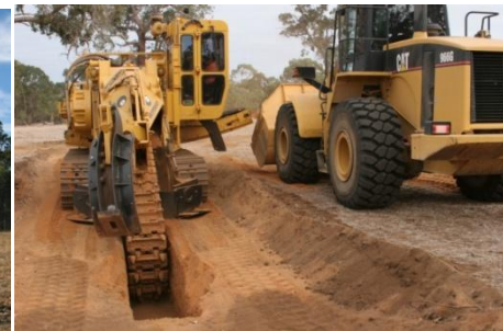
BRL's Sample Trench Drilling
