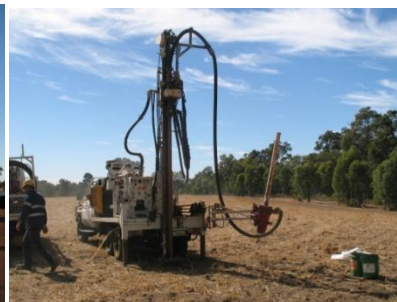
BRL Contractor Vacuum Drilling
