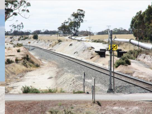
Potential available infrastructure (rail, electricity, water)
