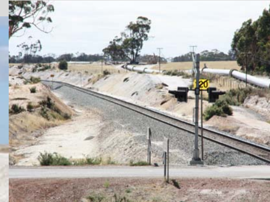
Potential available infrastructure (rail, electricity, water)
