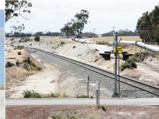
Potential available infrastructure (rail, electricity, water)
