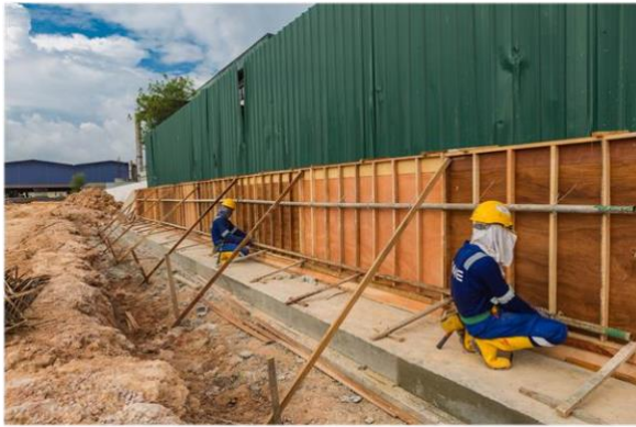
Boundary retaining wall
