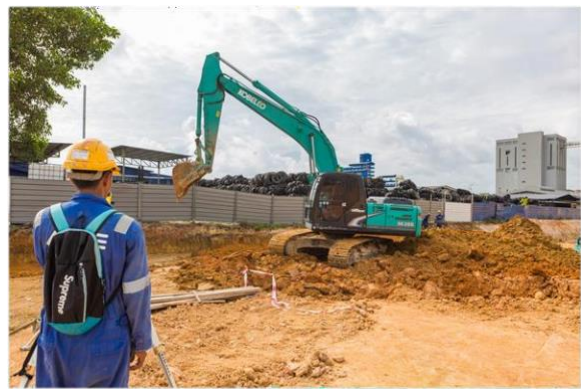
Workshop building ground works
