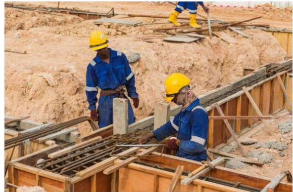
Building civil footings
