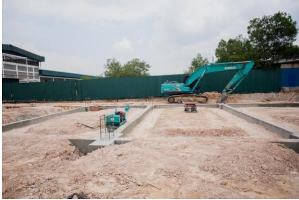
Building concrete footings
