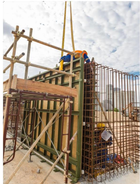
Steel work for concrete retaining wall
