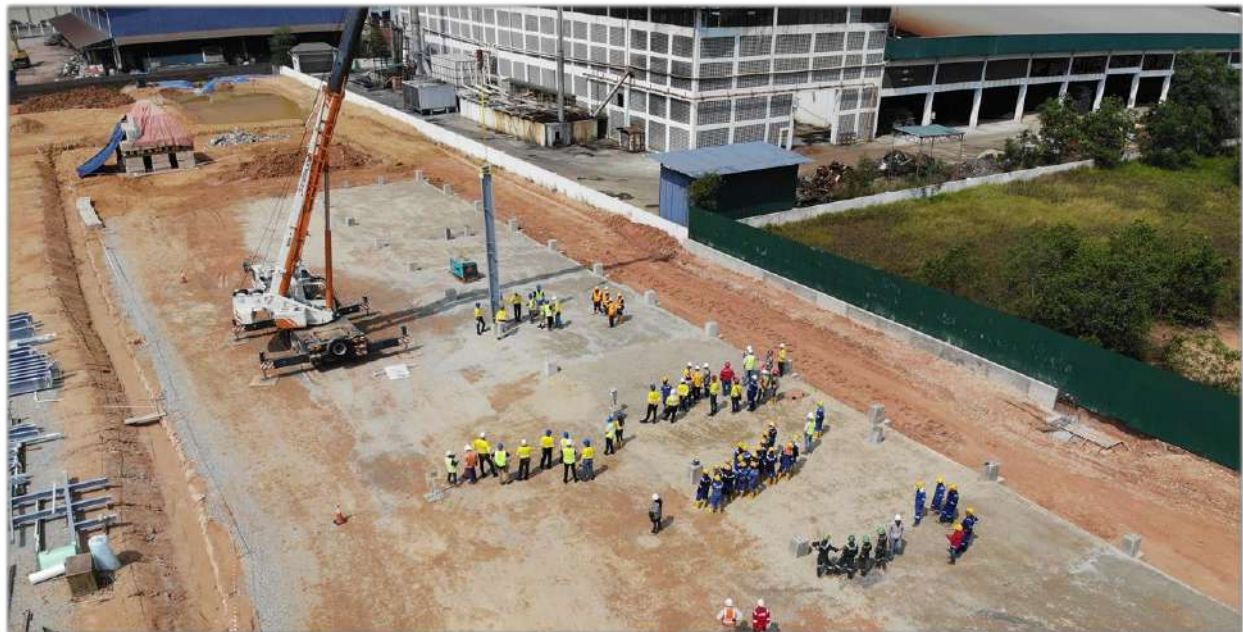
Erection of the first maintenance workshop column
