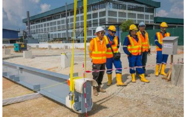
First steel column ready for lift
