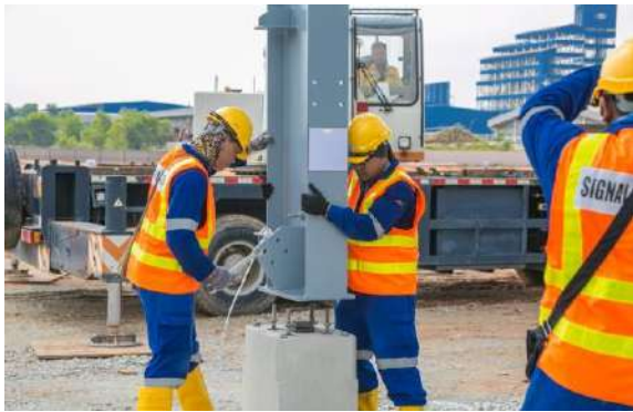
Securing the first steel column
