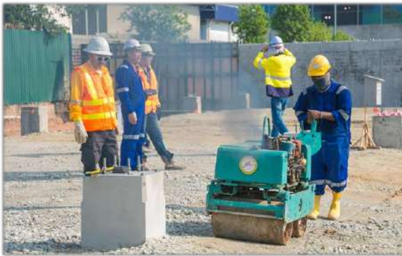
Concrete footings of workshop building
