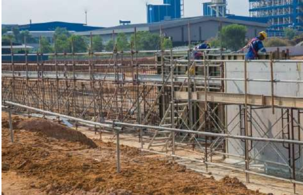
Administration building retaining wall
