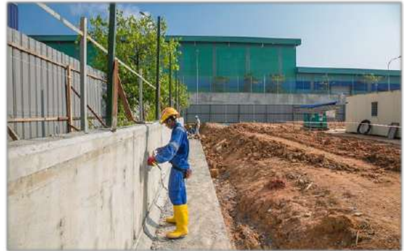
Boundary retaining wall
