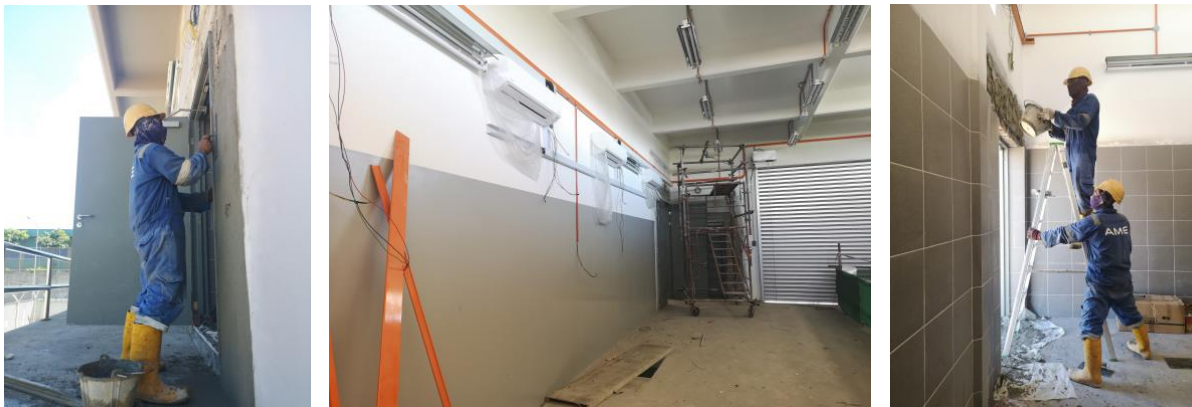
Photos - Construction work recommences at Altech's HPA site
