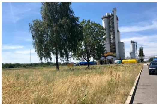
Front of AIG's industrial site
