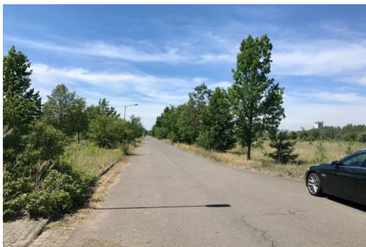
Internal roadway accessing AIG's industrial site
