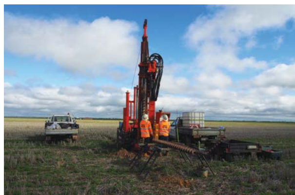
Astron Donald Project site geotechnical drilling (2021)
