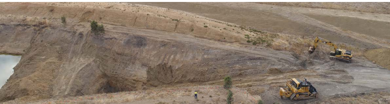
Donald Mineral Sands' Project excavation test pit.
