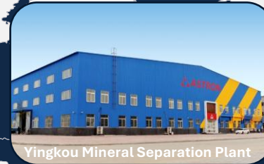
Yingkou Mineral Separation Plant
