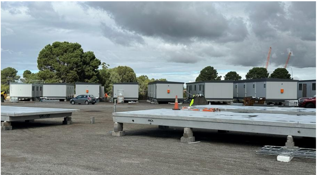
Ausgold accommodation modules at ADD's Perth facility
