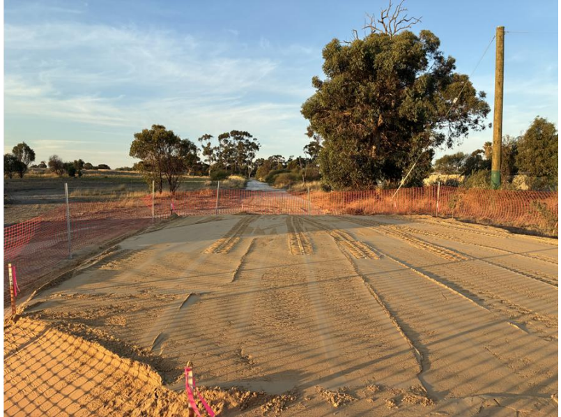
Site works for installation of electrical supply
