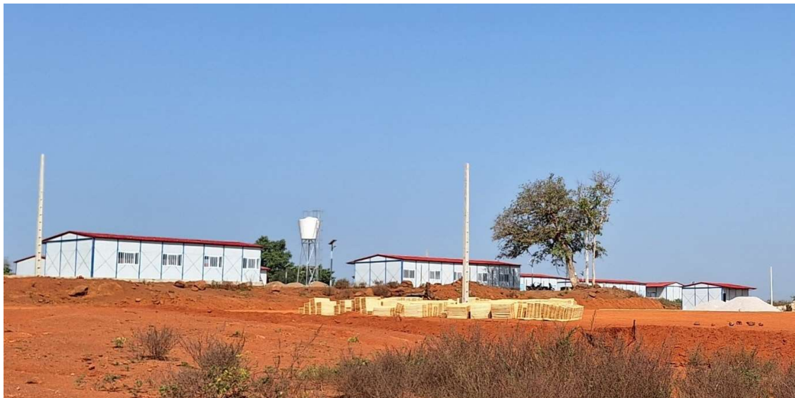
Figure 1 Newly built central exploration camp for Boundiali Gold Project
