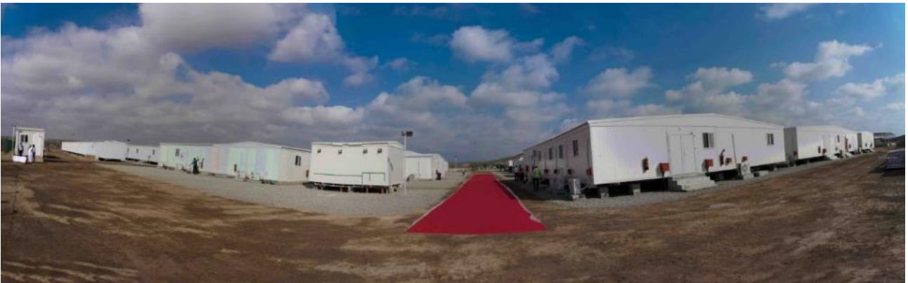
Accommodation village (wide-angle view)
