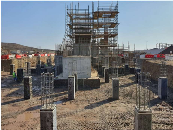
Mill area platform column foundation works
