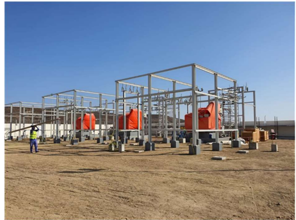
Primary substation - electrical works in progress
