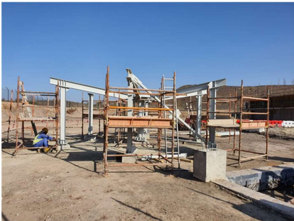
Copper concentrate thickener erection in progress
