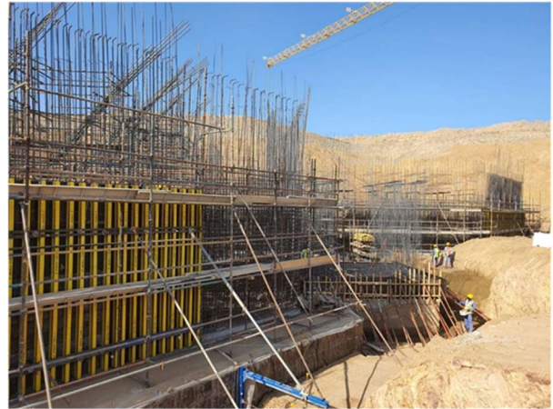
Primary crusher house under construction
