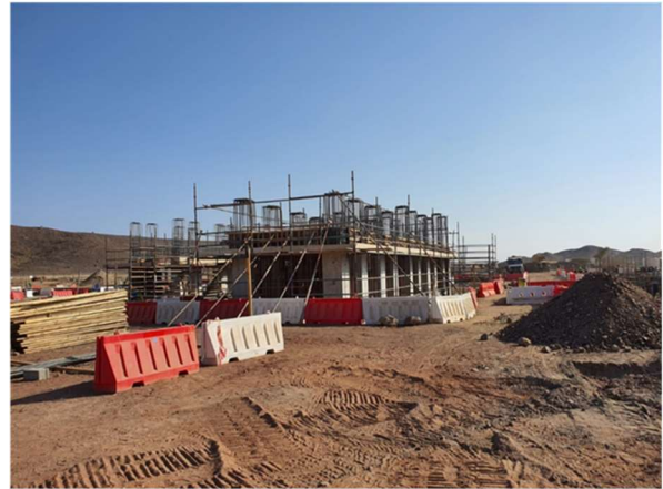
Rougher flotation cell foundation works
