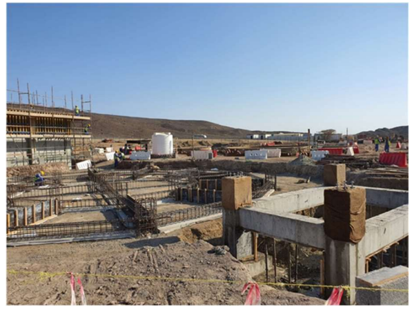
Tailing thickener backfilling works in progress
