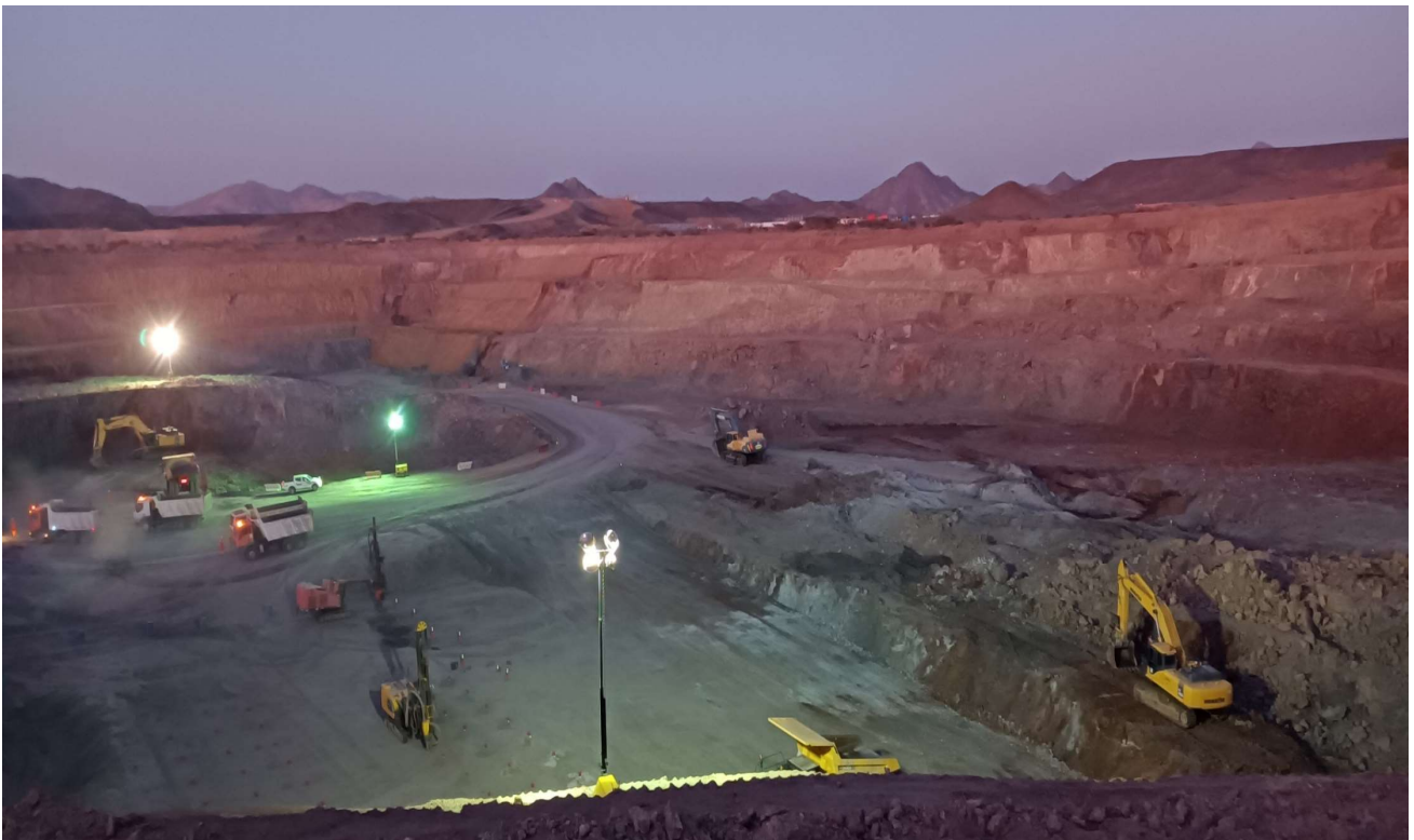
Night mining works
