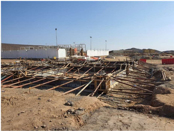
Bulk reagent storage under construction
