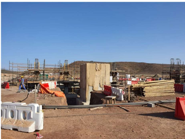
Regrind mill foundation works
