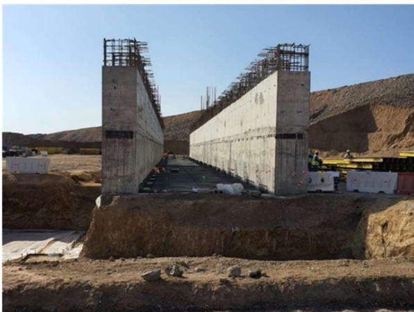
Crushed ore stockpile side walls completed
