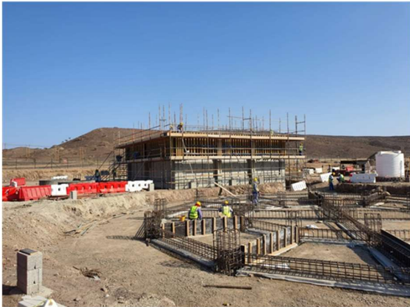
Concentrate filter house & storage yard
