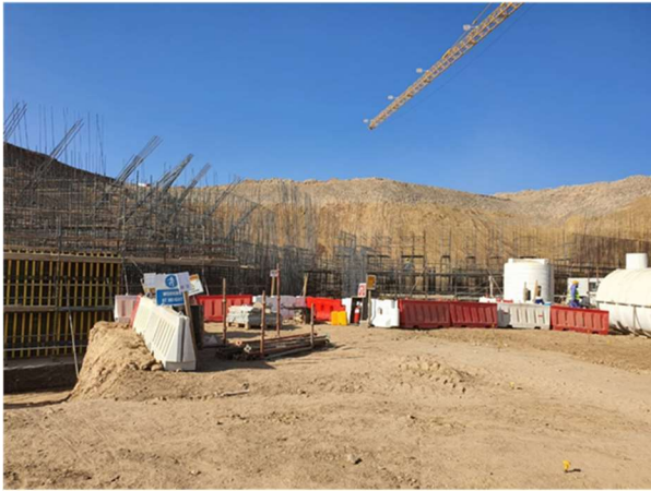
Primary crusher retaining wall under construction
