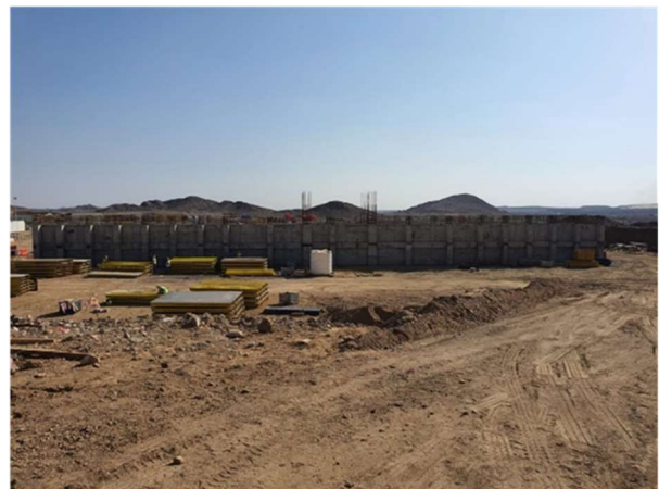
Roof slab under construction
