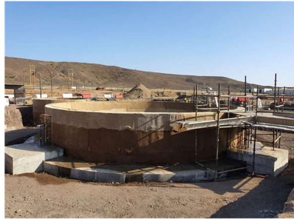
Tailing filter tank foundation
