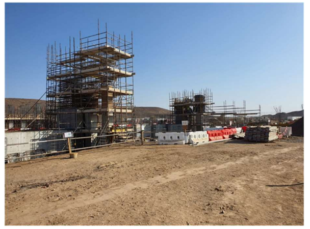
SAG and ball mill housing works
