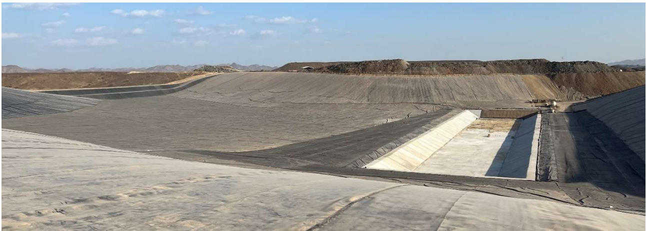
Image: Dry Processed Tailings Storage Facility
