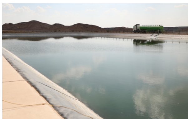
Fresh water storage facility
