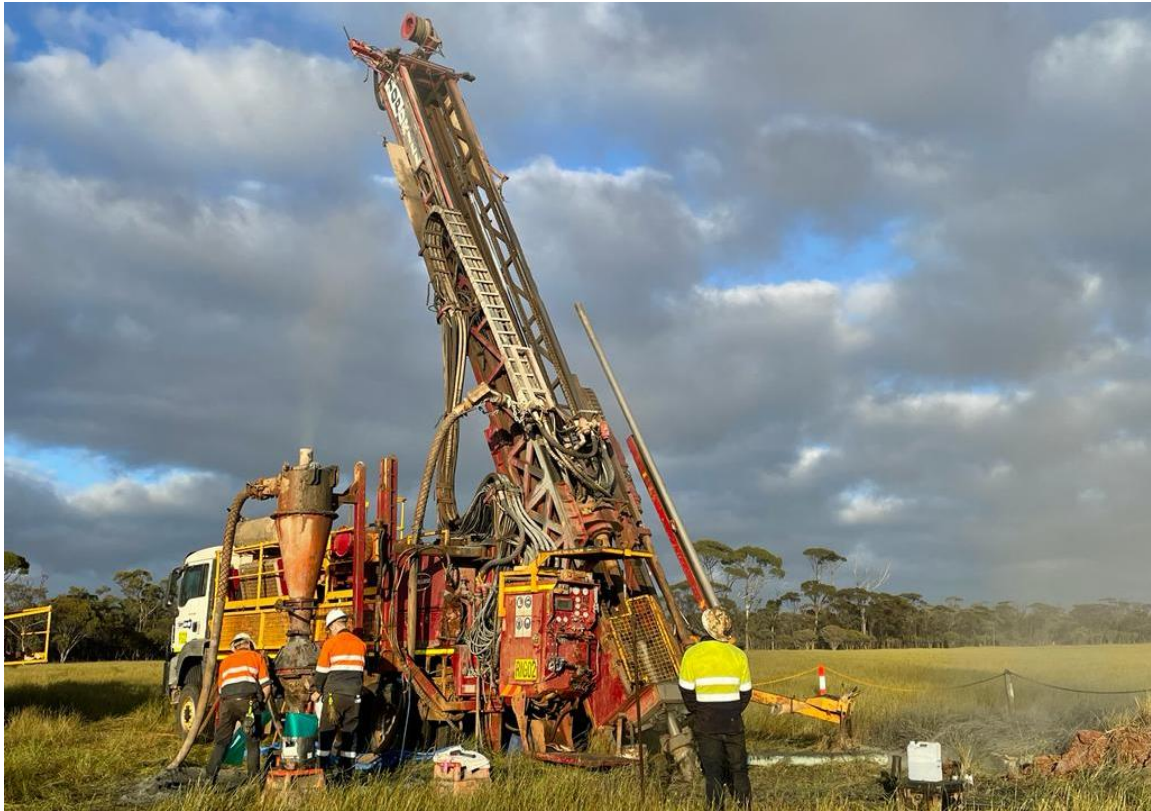
Figure 4: RC drilling in progress at Skeleton Rocks
