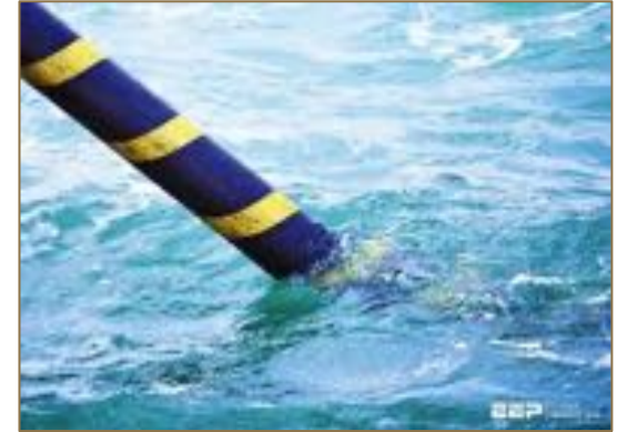
Sub-sea Power Cables
