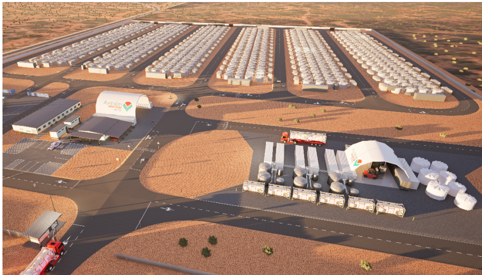
Figure 1: Conceptual render of a potential 50MW / 10-hour (500MWh) vanadium flow battery configuration for the proposed Kalgoorlie VBESS project
