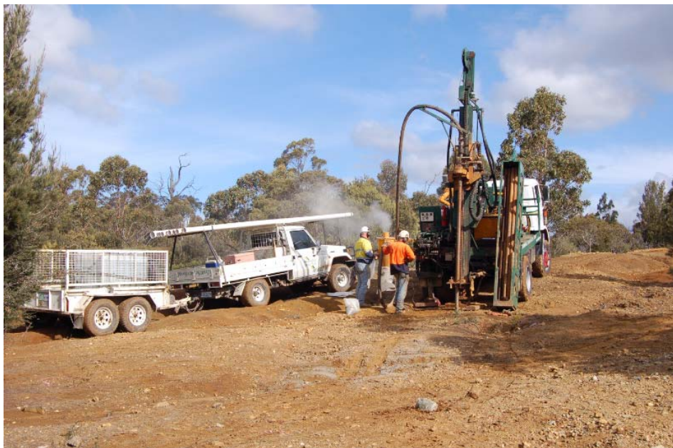
Figure 3: Barnes Hill Drilling
