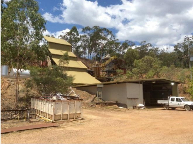
Photo 14/10/14 showing treatment plant at Mount Veteran
