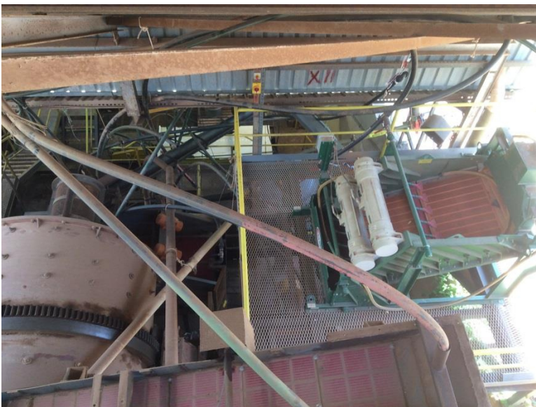
Photo 14/10/14 Mount Veteran Plant from crusher
