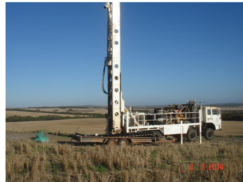
Campoona Shaft auger drilling
