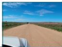
Jamieson Tank Road (looking east)
