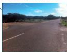
Cleve-Kimba Road junction with Elson-Campoona Road (looking north)
