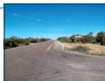
Cleve-Kimba Road junction with Jamieson Tank Road (looking south)
